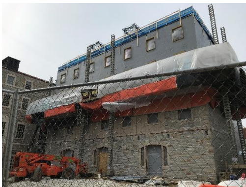
Continued Construction – New Addition
